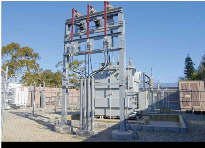
The 12.47-kV side of the new University of California, Santa Barbara-owned 20-MVA 66/12.47-kV substation.
