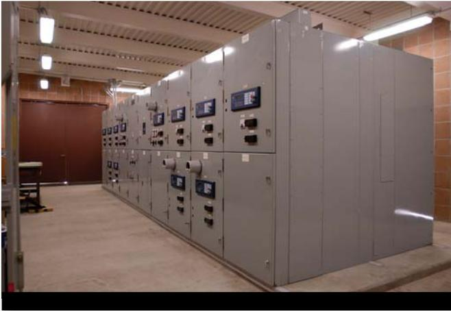
New switchgear building with new indoor vacuum circuit breaker and metal-clad switchgear.
