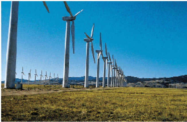
Foot Creek Rim, a 69 unit wind project provides a combined output of more than 40 MW to the power grid.
