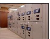
Though many secondary switchboards have outlived their service expectancy, Phase 1 did not allow for their replacement. Consequently, internal building utility upgrades are planned for the future. Phase 2 will continue conversions from 4,160- and 16,000-volt primary transformers to 12.47 kV. Two more 12.47-kV loops will be installed with eight interrupter switches and 5,000 ft. of ductbank. Furthermore, 10
